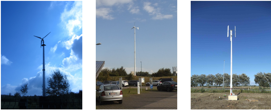
Figure 2.3: Wind turbines purchased, installed and tested for this dissertation.
